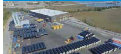
XXL PIPE PRODUCTION FACILITY CHARLESTON, SC/USA
